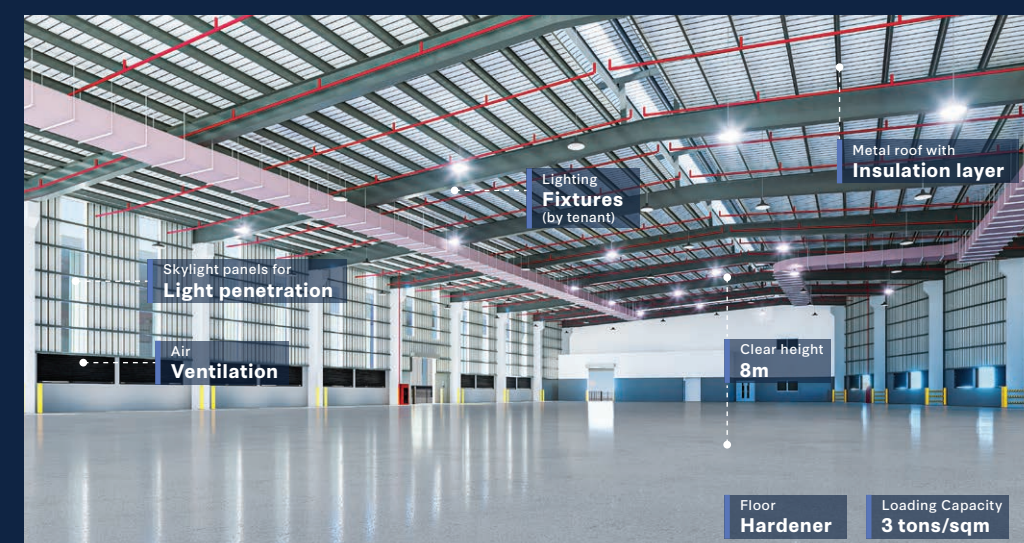
Ready-built Factory | Ground Floor
